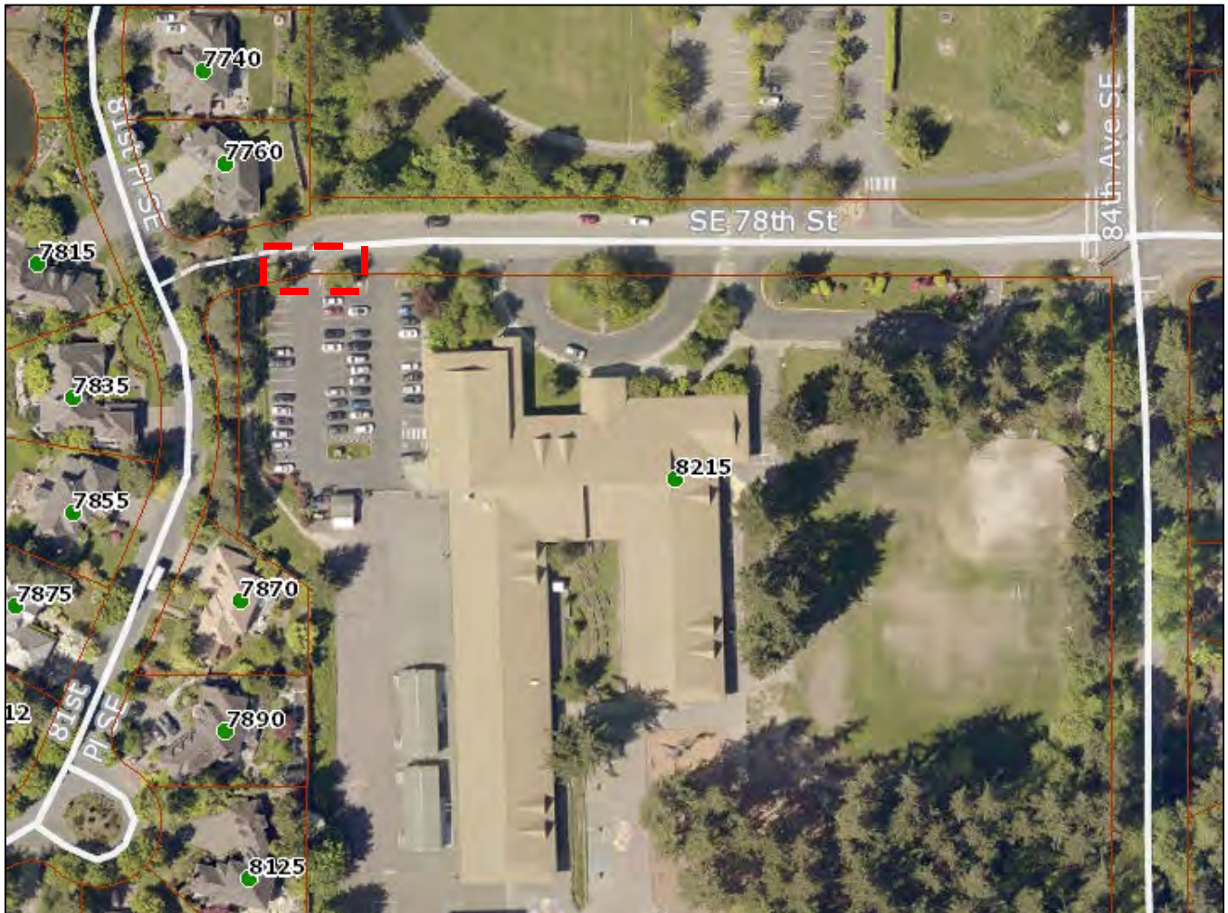
Project Area with four subject trees outlined with red dashed rectangle, Lakeridge Elementary School is southeast of project site; King County Parcel Viewer aerial image
